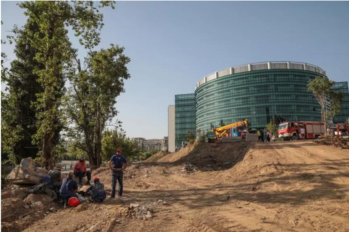
Image 1. The construction site where the accident occurred
